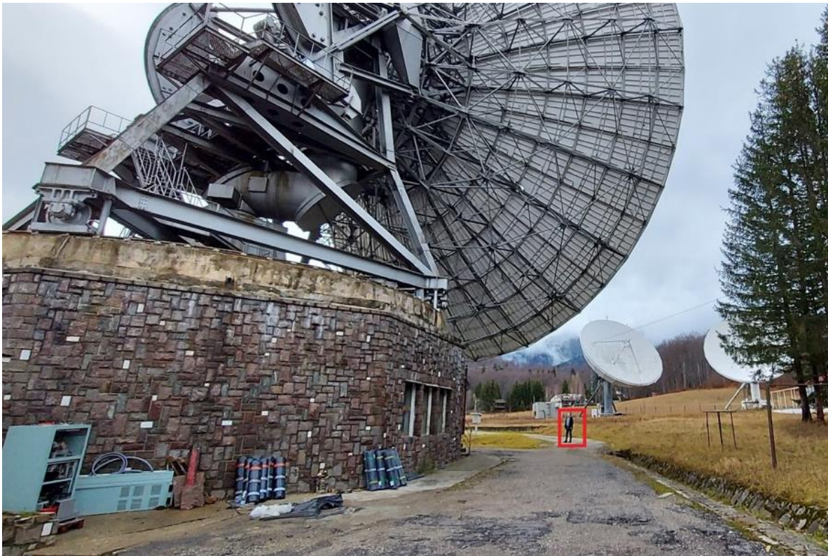
Figure 146. Cheia1 RADAR's antenna (32 meters wide, 309 tons of weight)
